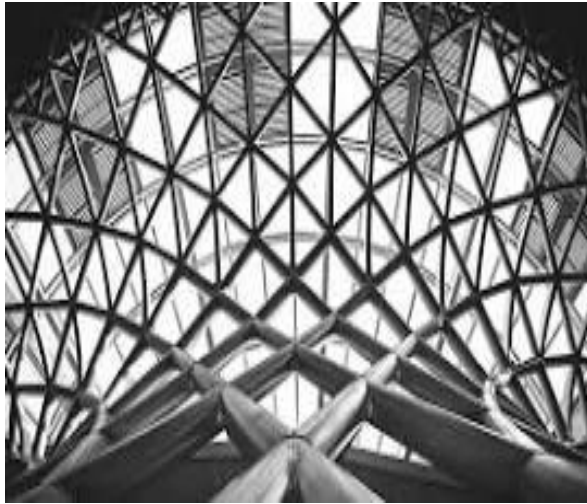
Fig 1: Diagrid Structural System
