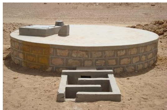
Figure1.2: Tank Resting on Ground
