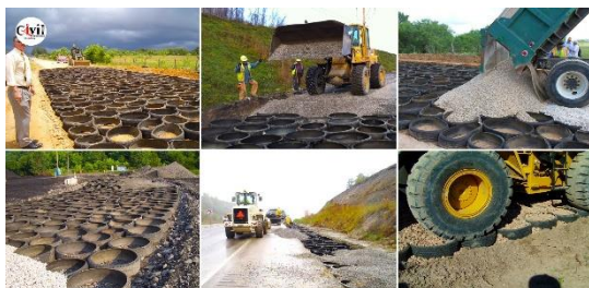
Figure no. 3:- using waste tyres in road construction
