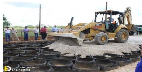
Figure no. 4 :- waste tyres in road construction
